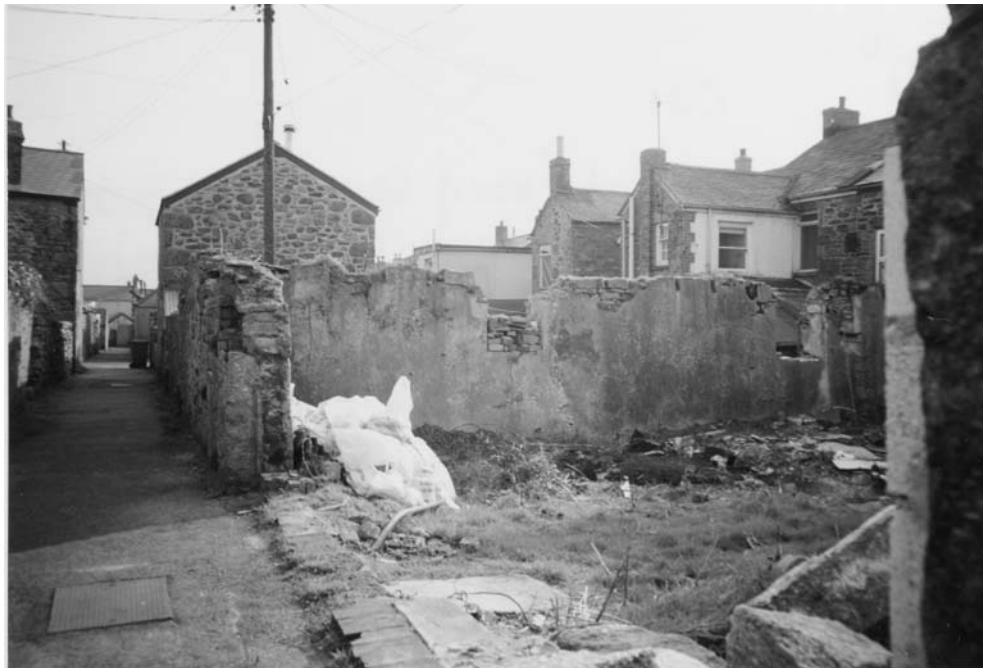
Figure 10 The rear yards and alleys of St Just retain a large and important number of original yards, outbuildings and walls that define the character of the town more
