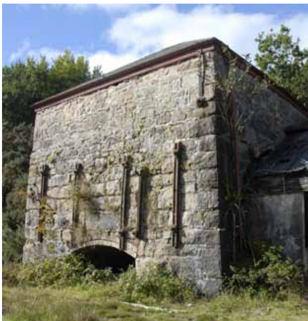
Above: The Tolgus Calciner near Redruth, a Scheduled Monument and the most complete example of this rare ore dressing structure
