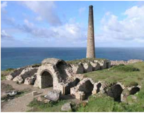
Above: The restored arsenic labyrinth at Botallack Mine, West Penwith
